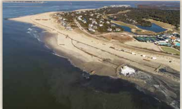
Aerial photo of sand placement on South Beach from the Army Corps of Engineers' Wilmington Harbor Inner Ocean Bar Project.
